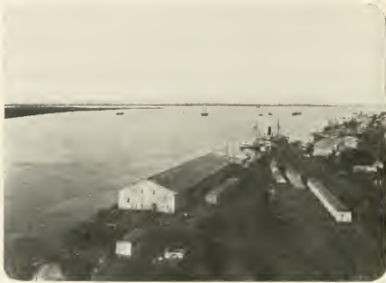
River Paraná from Grain Elevator.
