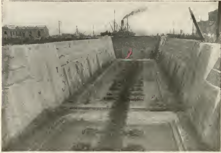
The Dock, Keel and Bilge Blocks.
