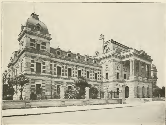
Water Works Building.
